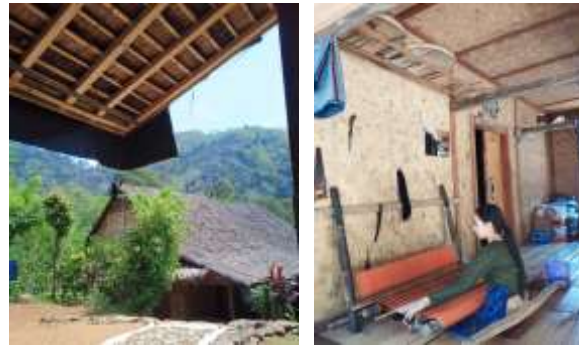
Figure 1. The roof of the outer Baduy house (left); wall and floor of Baduy house outside (right) on Baduy Luar
