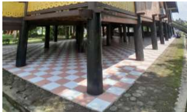
Figure 1. Supporting pillars of the Kajang Lako Jambi Traditional House
