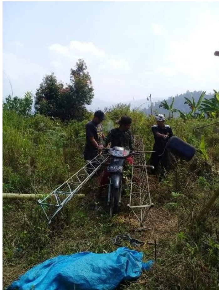
Figure 11: The Struggle to Carry a Tower in the Forest.
