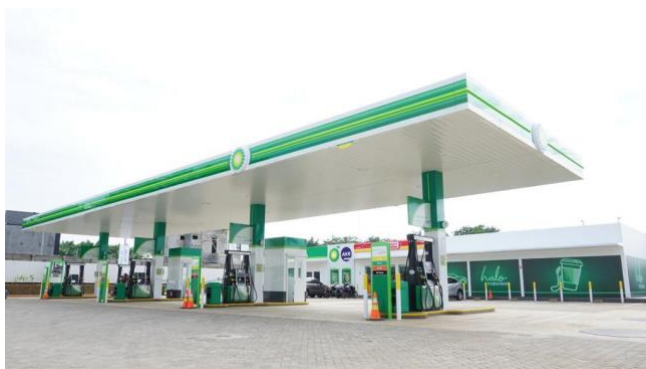
BP-AKR's Gas Station
