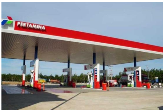
Pertamina's Gas Station
